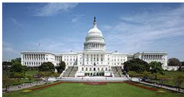
The West Front of the United States Capitol (begun in 1793.) Its 'wedding cake' cast iron dome draws heavily from the Renaissance dome of St. Peter's Basilica in the Vatican
